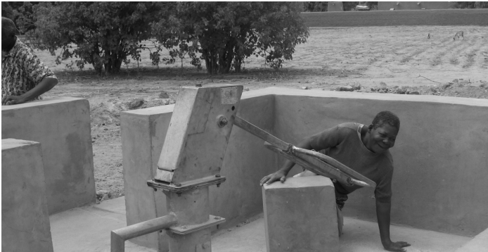
Cecile, who does not have use of her legs, climbs onto the concrete seat that our team installed at the pump testing site.
