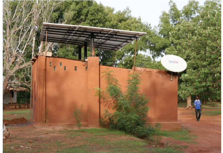
VSAT dish mounted at corner of the battery shed in Mahadaga for satellite Internet connectivity.
