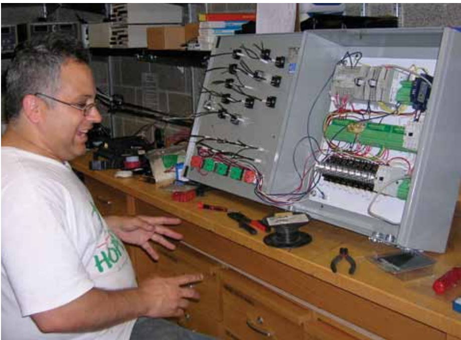
Engineering Student Philip Martinez '12 works on the automated biodiesel processor control panel.
