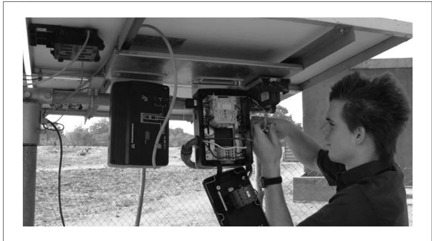
Matt Rooke '05 wiring the pump.
