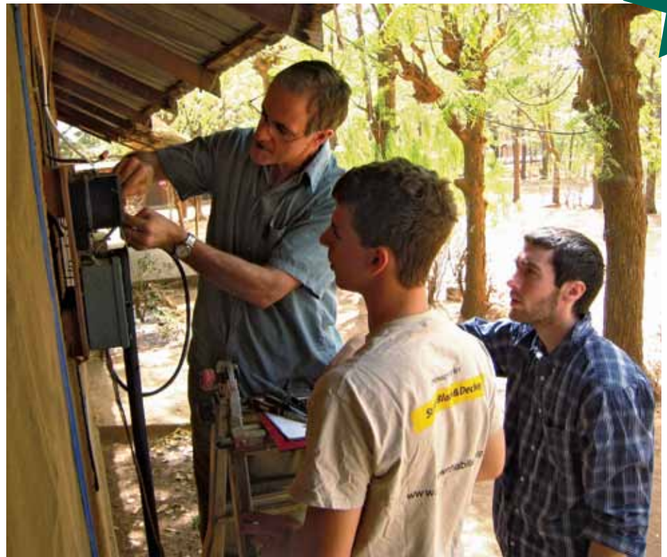
Professor Randy Fish (left), Kevin Manieri '12 (center) and David Allen '12 (right) install a kilowatt hour meter at the Center for Advancement of the Handicapped (CAH) in Mahadaga, Burkina Faso.
