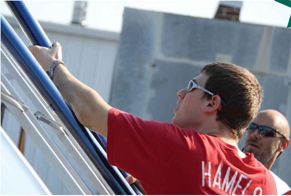
Andrew Dowling '13 (left) installs solar evaporated tubes on the roof of the Hess/Miller Residence for the solar hot water heaters that were installed last year.
