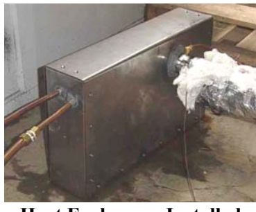
Heat Exchanger Installed
