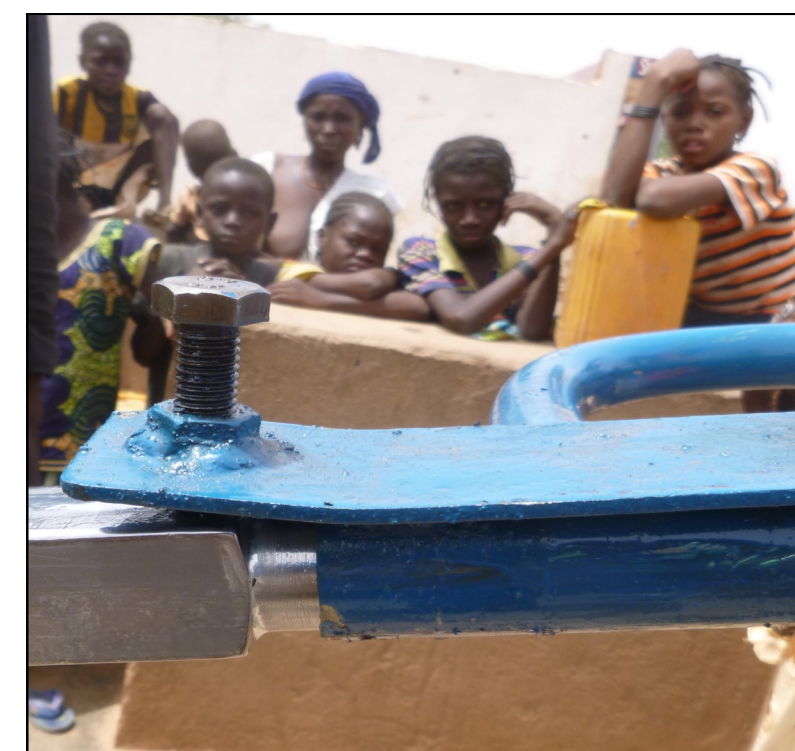
Failed modified pump handle in Niger due to high force.
