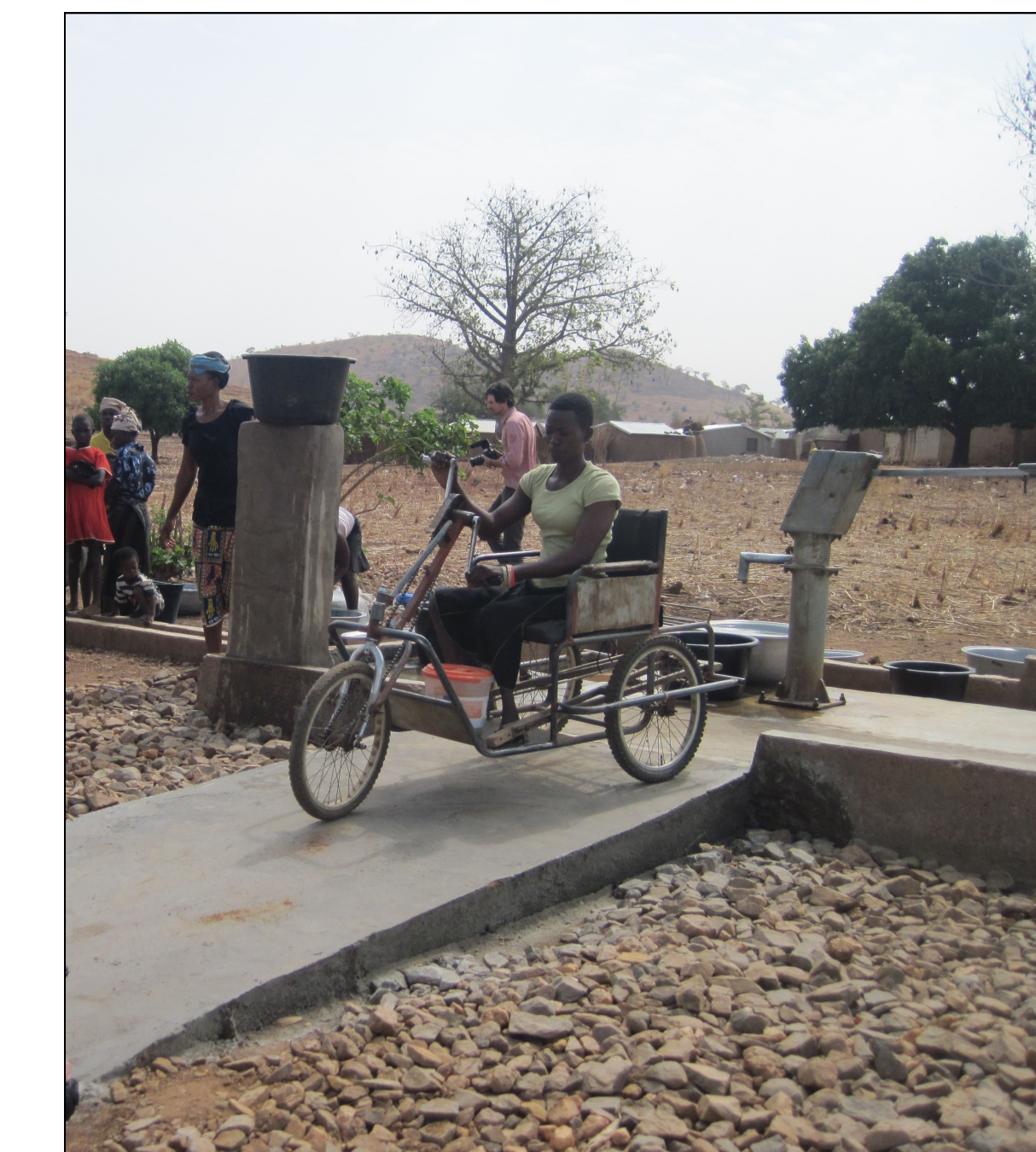
Above: A woman using a modified pump superstructure to fetch water from a tricycle.
