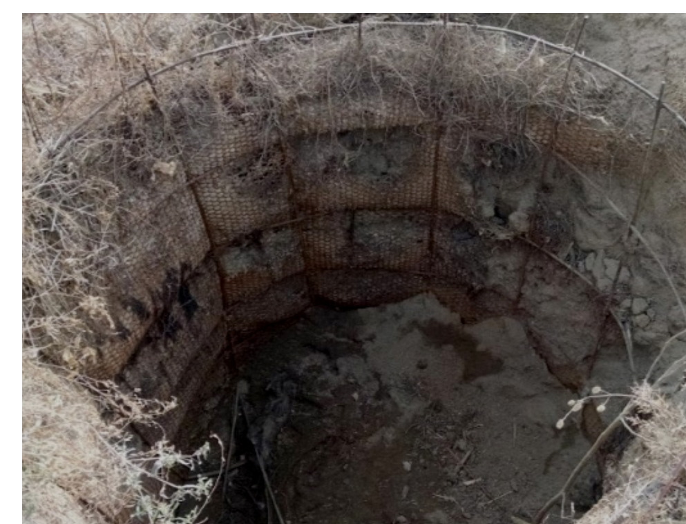
The rebar reinforced fabric liner from 2016
