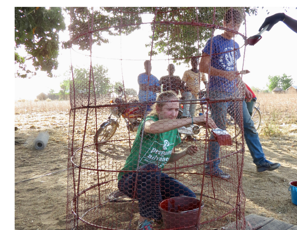
One of the modifications of the design was painting the rebar and chicken wire, as seen in the photo above.
