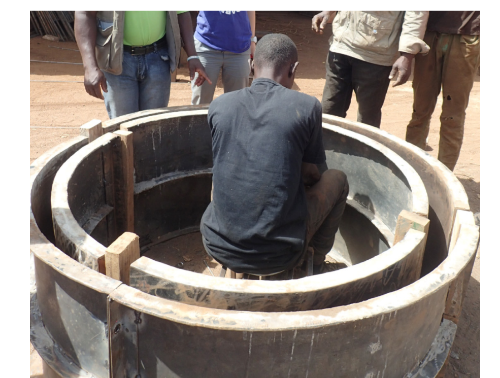
The modified ferrocement mold
