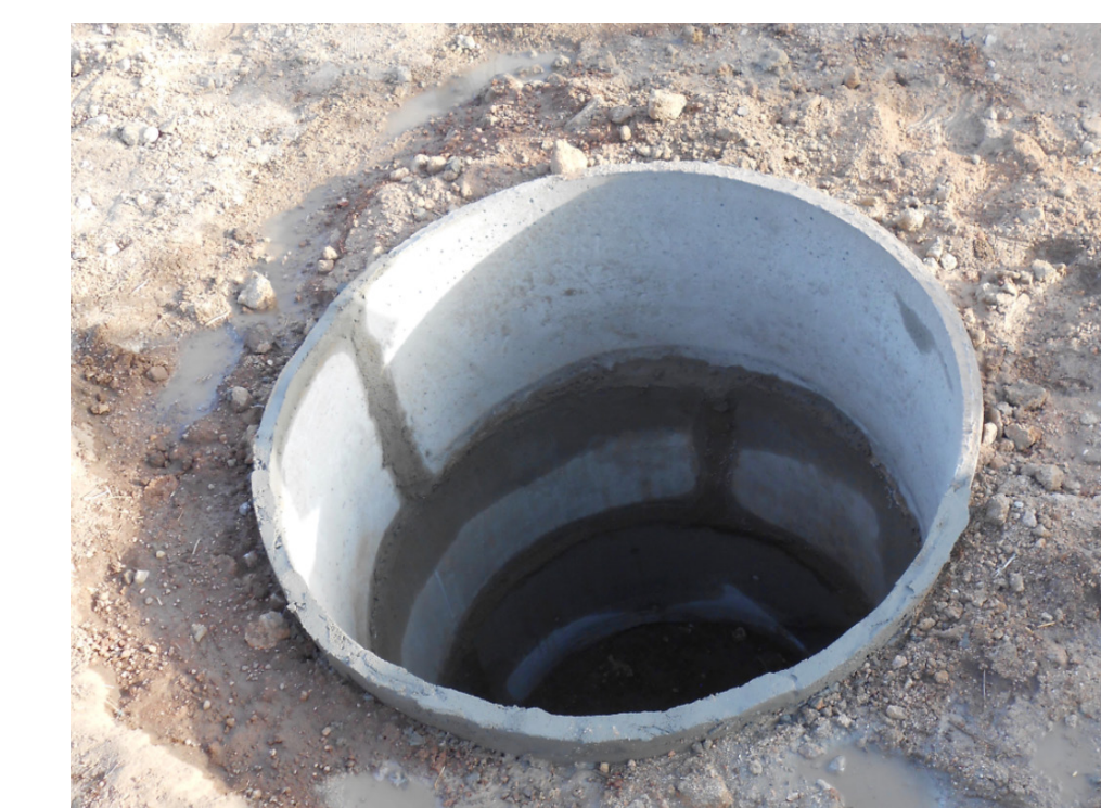
The completed ferrocement liner
