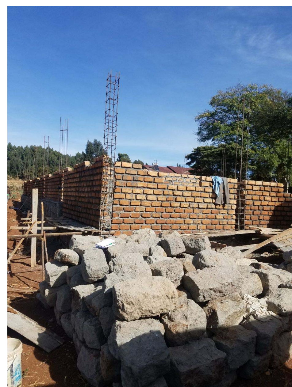
Figure 5: Pamajo Hall Being Constructed (Feb. '18)
