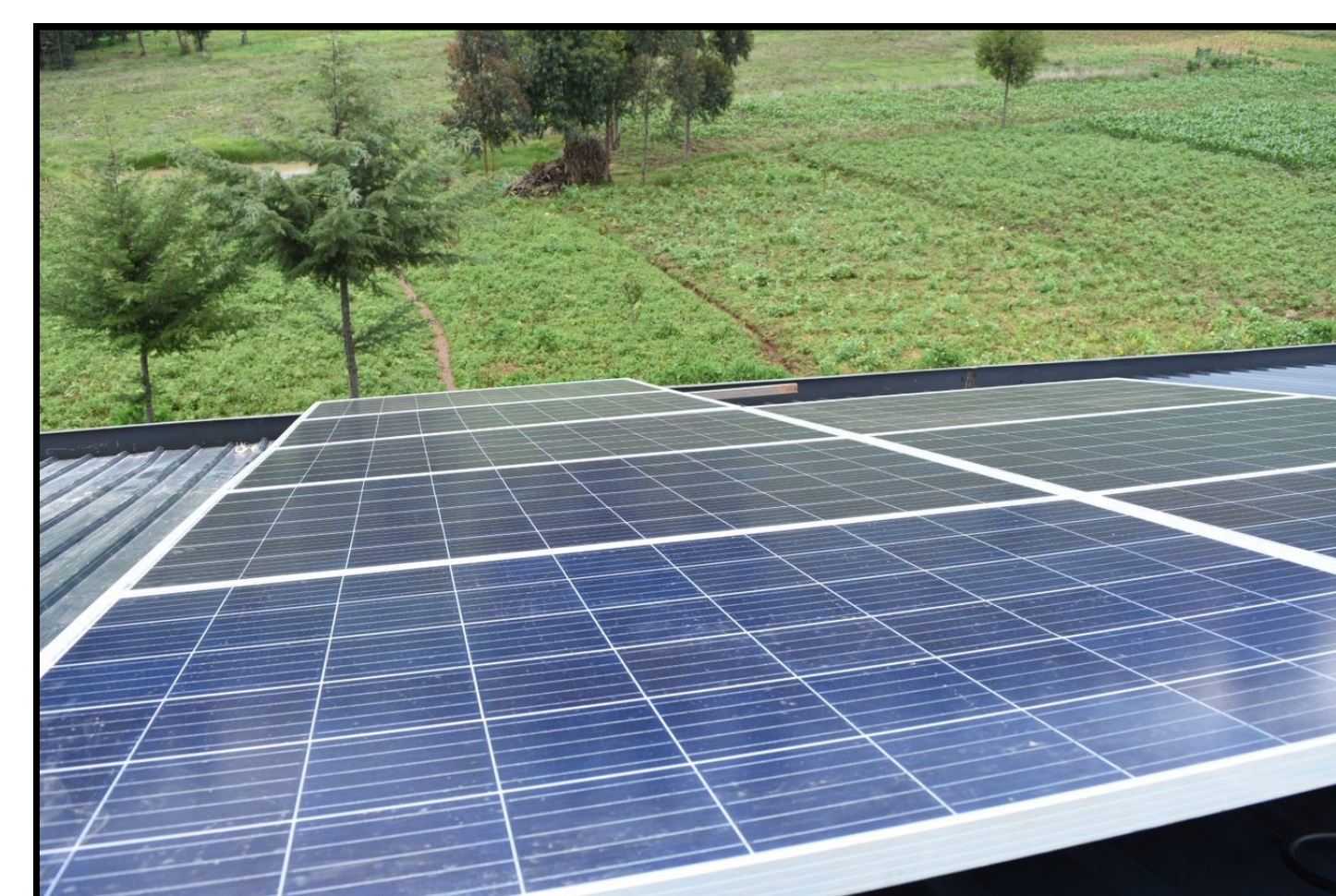
Figure 5: Panels on Roof of Pamoja Hall—Summer 2018
