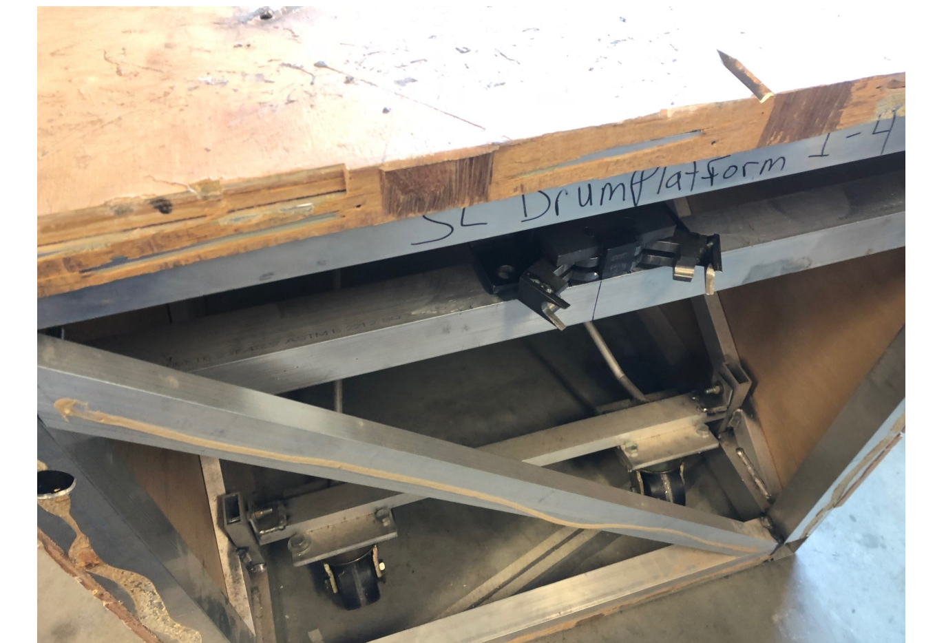
Latch installed in sample set piece
