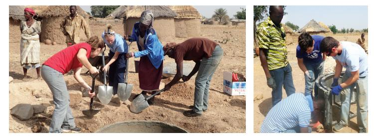
Above left: Rachel Aukamp '18 and Cheylee Smith '20 dig around the newly implemented ferro-cement liner to create a level ground surface for laying the concrete slab. Above right: Eric Denlinger '19 and Adam Barley '19 remove the ferro-cement liner from its mold.
